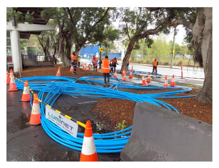
The 6912F cables used are from AFL and feature Fujikura's patented SWR® Spider Web Ribbon technology and 12 fibre MPO FUSEConnect® terminations to give flexibility on fibre distribution points within each Data Centre.
